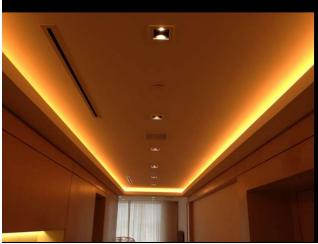
120 Leds/m - DC12V & 24V - 8mm - 9W/m RA 80 - IP20
